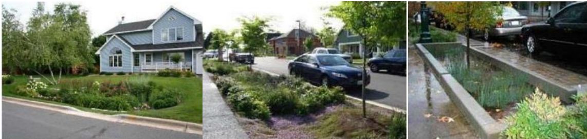
Figure 16. Three examples of curbside stormwater solutions, referred to as rain gardens, bio swales and bio retention cells
