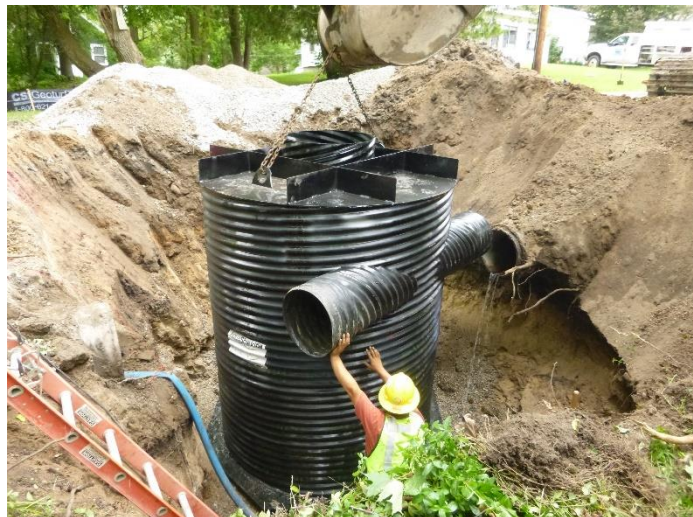
Figure 14. Oil/grit separators use various approaches to separating solids that settle at the bottom of the unit and oils and trash that float to the top. These pollutants can then be removed and disposed of properly. Water is allowed to pass through. Water soluble pollutants such as fertilizers and salt are not treated.
