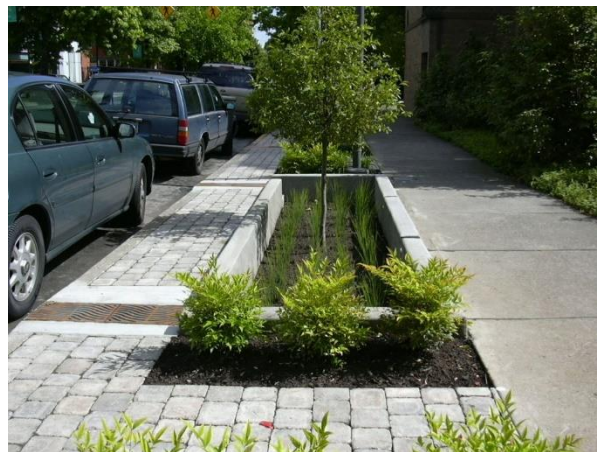
Figure 19. Tree trenches can increase holding capacity and infiltration in developed areas. Above ground they look like typical city trees.
