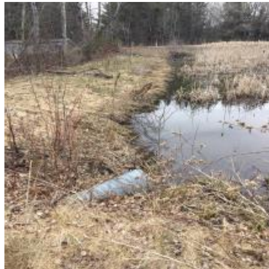
Figure 15. This is an example of a wet detention basin in Lewiston. The pipe pictured carries stormwater to its final destination in a retention basin. (Photo sourced from RLS, 2020)
